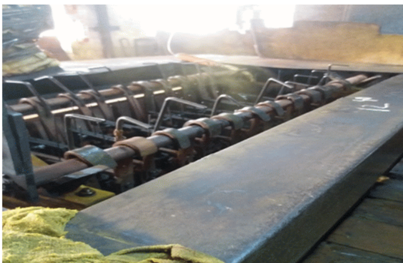
Fig. 1. Emissions in the form of vapors in the galvanic workshop
