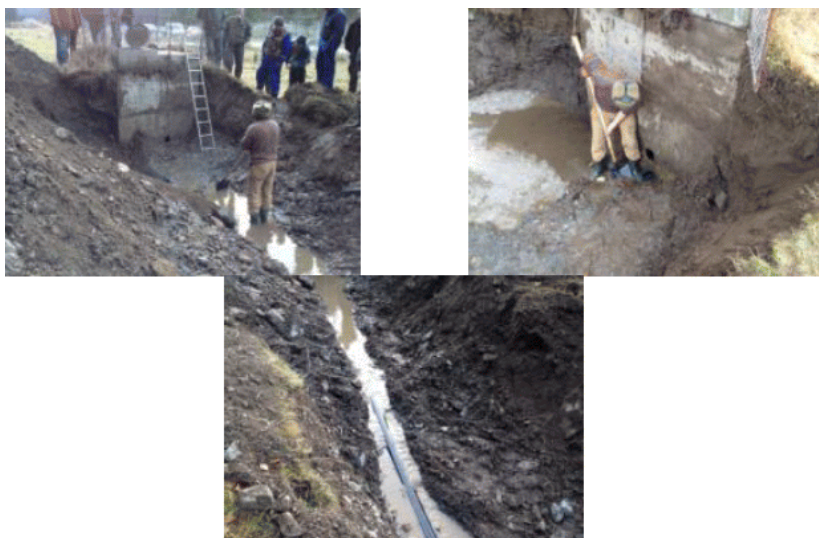
Fig. 2. Conducting surveys - mechanized excavation onsite
