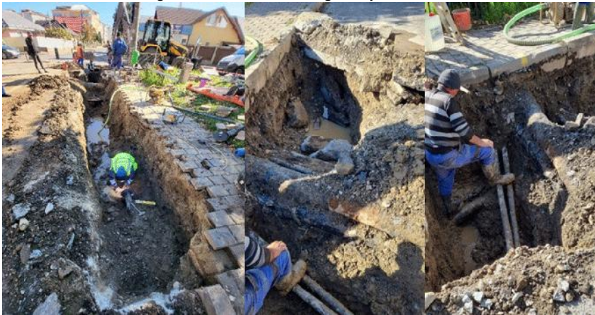
Fig. 7. Pipe replacement
