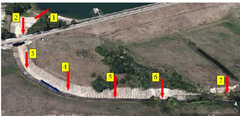
Fig. 4. General view of the high flow evacuator 1 - access channel; 2 - spillway; 3 - connection channel; 4 - inclined drop zone 1; 5 - inclined drop zone 2; 6 – hydraulic energy dissipater + downstream apron; 7 - escape channel (image Google earth)
