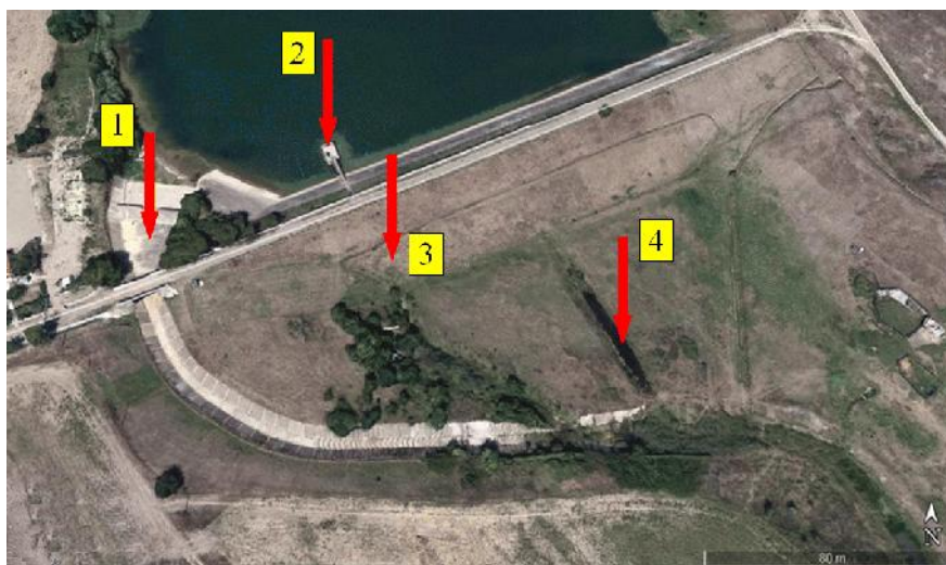
Fig. 3. General view of the location of the outlet structure at the Chiri a dam 1 - the high water discharger; 2 - manoeuvring tower and socket; 3 – unwatering conduit; 4 - sewerage drainage (Luca et al., 2004, image Google earth, 2010)
