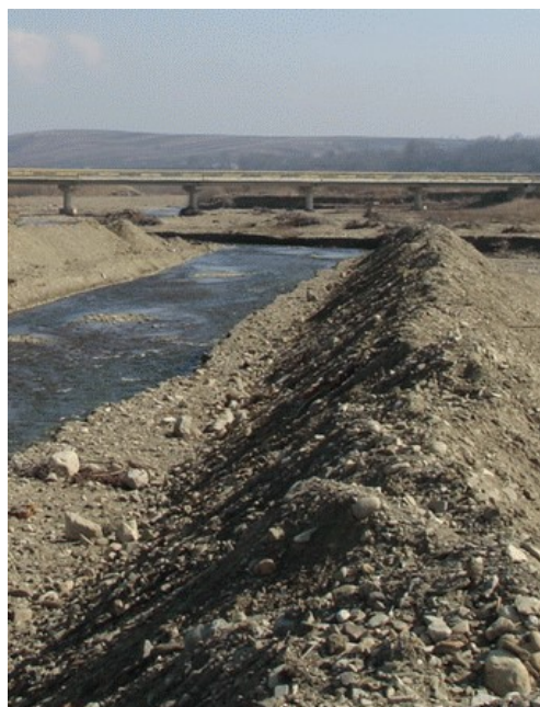
Fig 3. The reprofiled bed of the Tazlaur Sarat River in the research area (Luca M., 2017)
