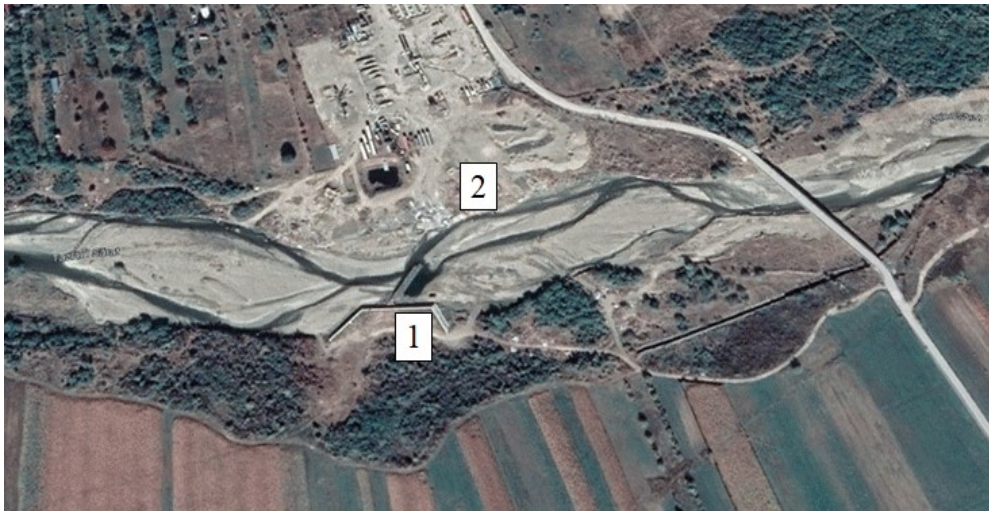
Fig. 8. View of the location area of the works carried out in the bed of the Tazlaur Sarat River at the eastern limit of the Moinesti city: 1 – protection of the bank with the location of the pipeline; 2 – the new bed of the river (sc. 1:100000 image Google earth 2023)
