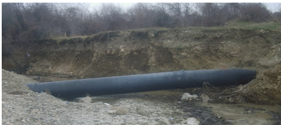
Fig. 5. The state of degradation of the adduction pipe site in the area of the bank right of the Tazlaul Sarat River from the outskirts of the Moinesti city (Luca M., 2017)
