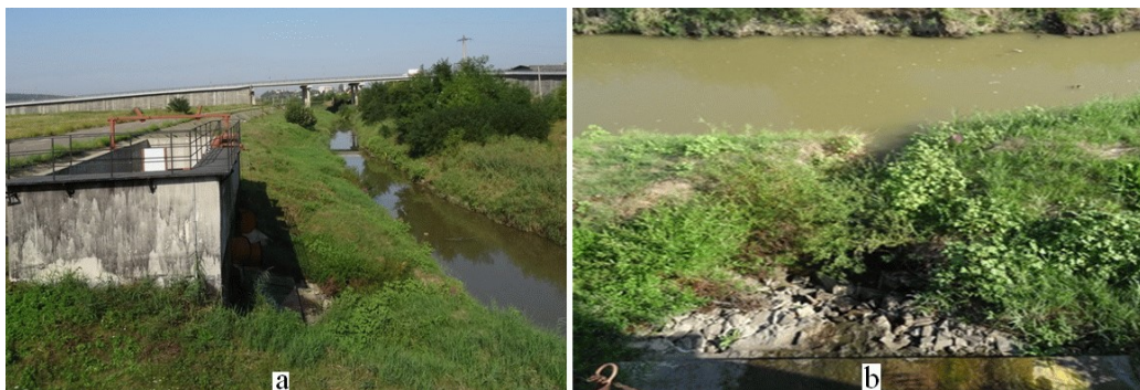
Fig. 8. Bahlui River bed interaction - right bank riparian area: a - rainwater storage tank and discharge with DC2 in the bed; b – overview of degraded structural states of DC2 (year 2019) (Luca M., 2019)
