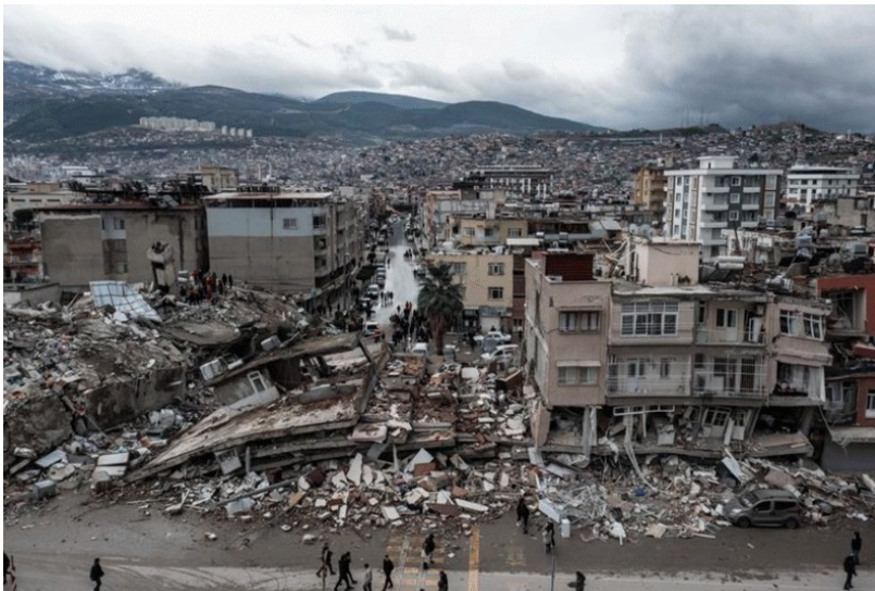
Fig. 2. The aftermath of the earthquake in Turkey[9]
